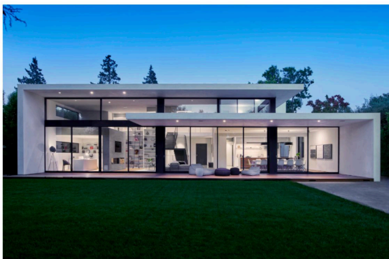
THE FLOATING BOXES HOUSE (CREDIT: JOHN SUTTON)
